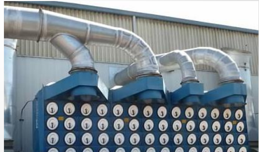
ventilation system directed to an Air Pollution Control Device
